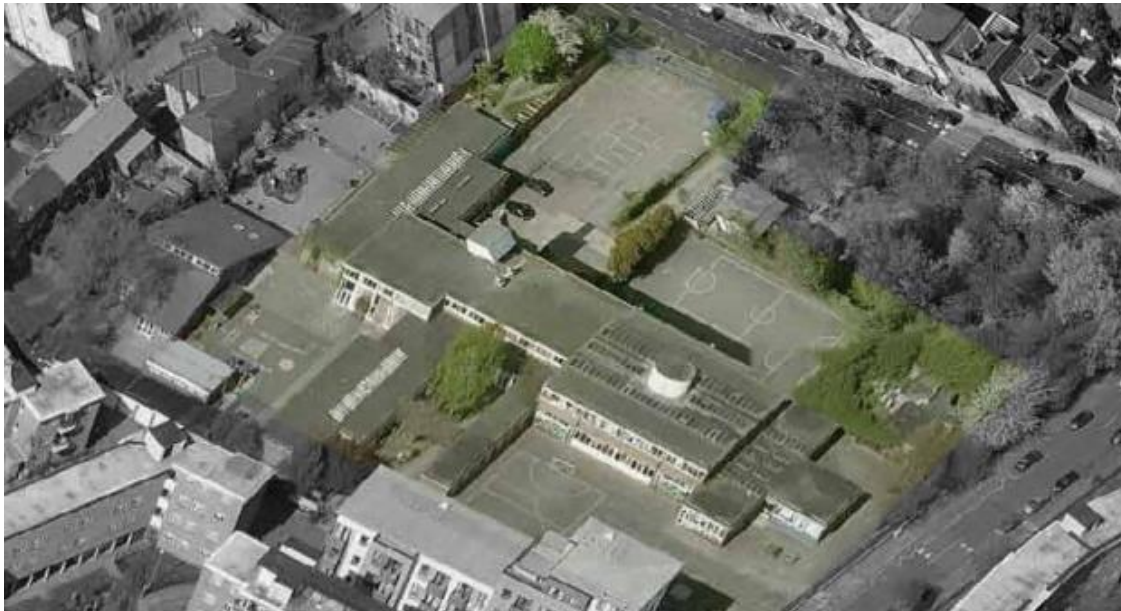
Figure.2 indicating the existing part one, part two storey school building
