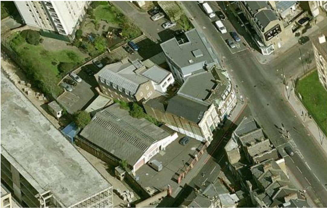
Fig. 1: Overview of existing site
