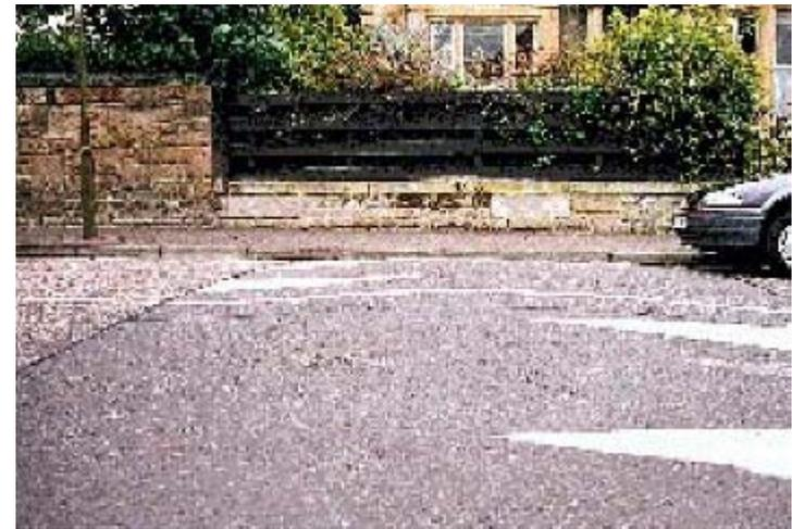
Warwickshire County Council used 75mm high flat-top humps with a similar rolled top ramp profile in the Rugby 20 mph zone. The average of mean speeds at and between the humps was 18 mph.
